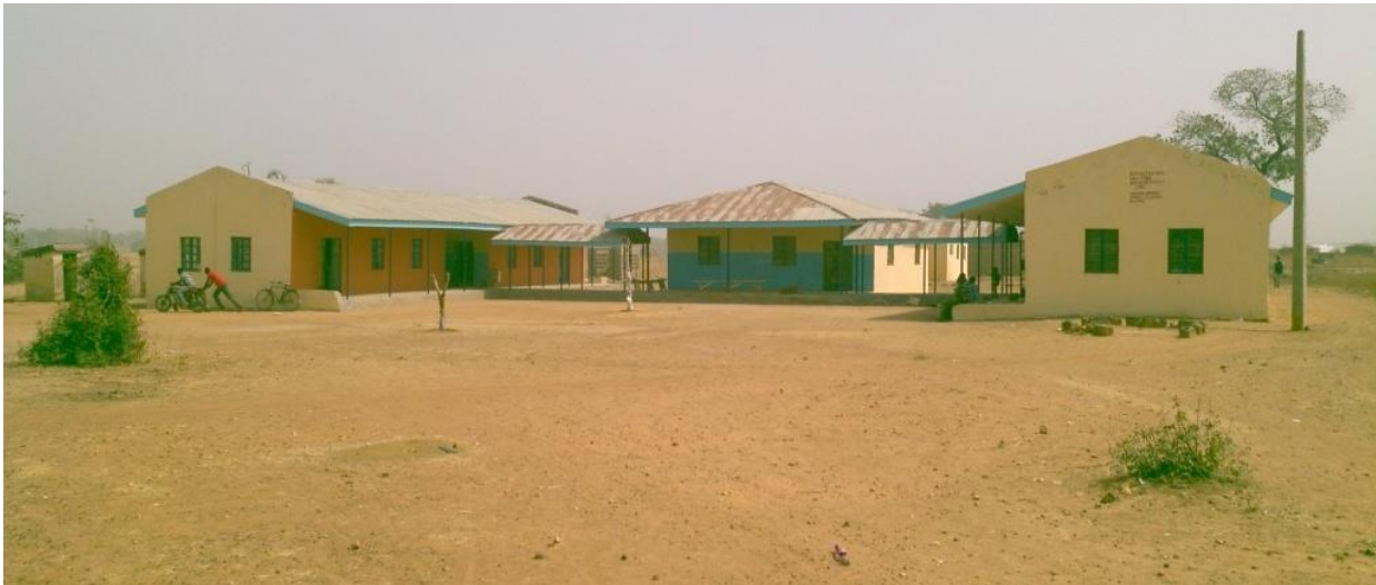
Fig 5: The Ministry of Health Clinic at Bagega, presently been refurbished by a GAVI supported fund
